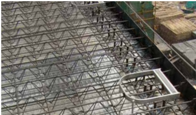
Special channel HCW 52/34: anchorage of high wind loads in thin slabs
