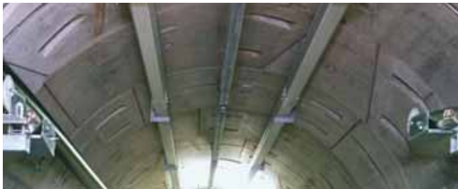
Curved HALFEN Cast-in channels in tunnel segments
