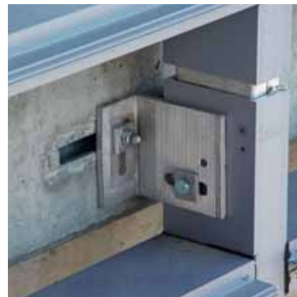
Mullion fixing at front of slab
