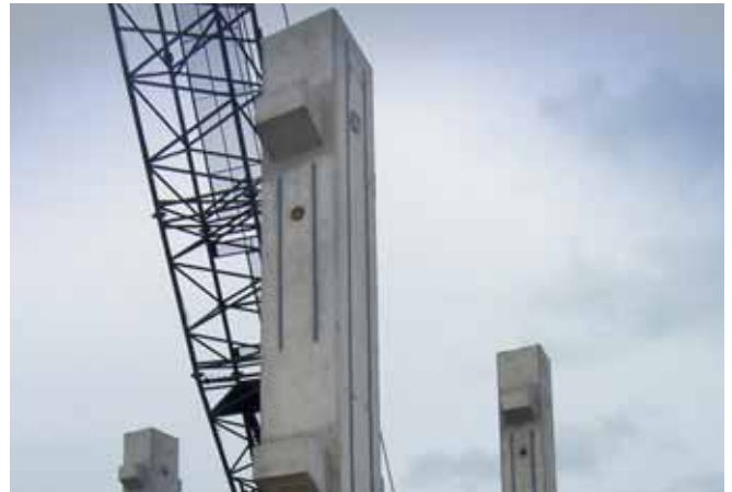
Vertically installed channels for pipe rack support
