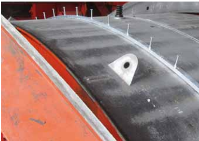
Channel installation into tunnel segment formwork
