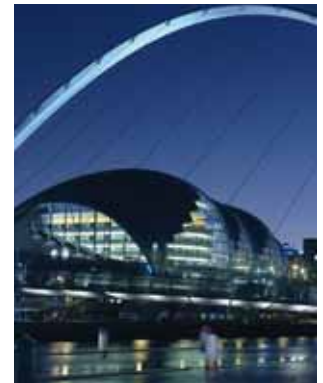
Sage Centre, Gateshead (UK)
