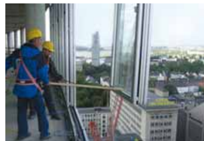
Modular panel installation
