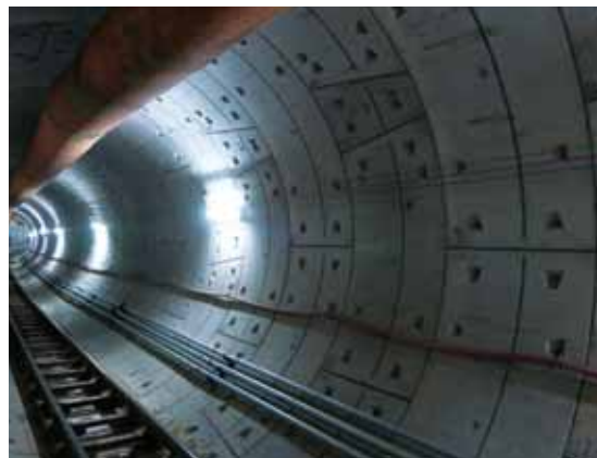
Curved channels in tubing segments, Shenzhen metro
