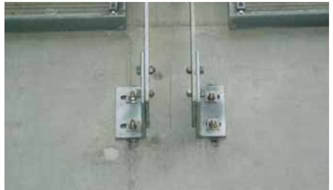
Custom-made brackets attached to vertically installed DYNAGRIP Channel pair
