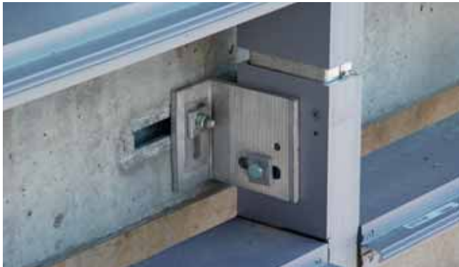
Mullion fixing using HCW-ED Brackets
