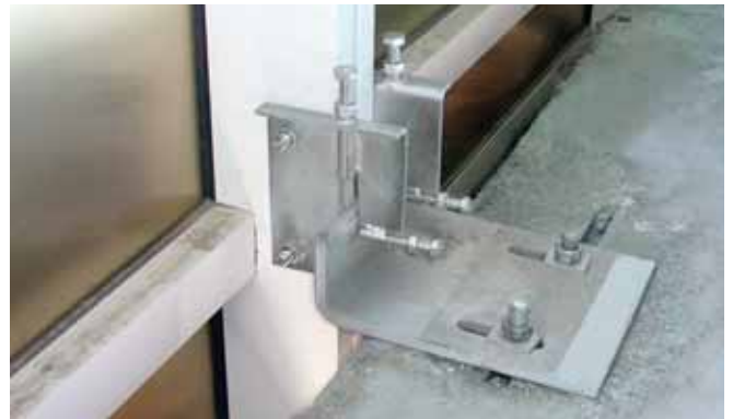
Fixing of curtain wall system using HCW-B2 Brackets connected to HTA-CE Anchor channels
