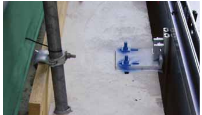
Top of slab fixing – colour marked for quality check
