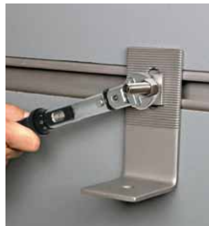
Tightening the T-bolt
